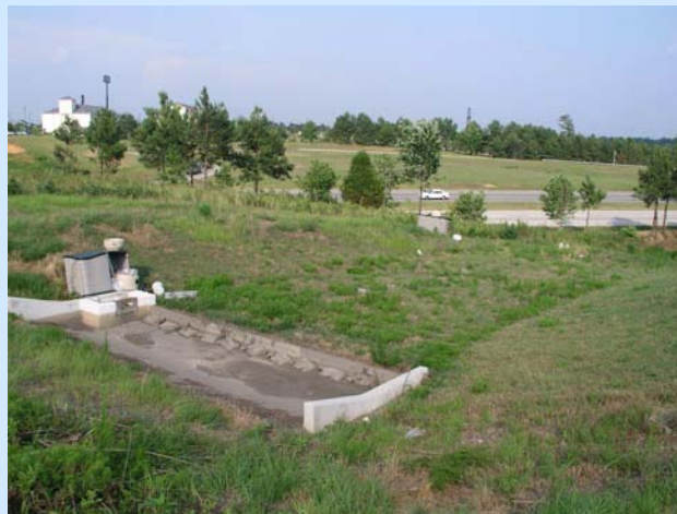
Figure 2.2-9: A filter strip that receives overpass runoff at Hwy 42 and I-40 in Johnston County, North Carolina (Wu and Allan, 2006).
