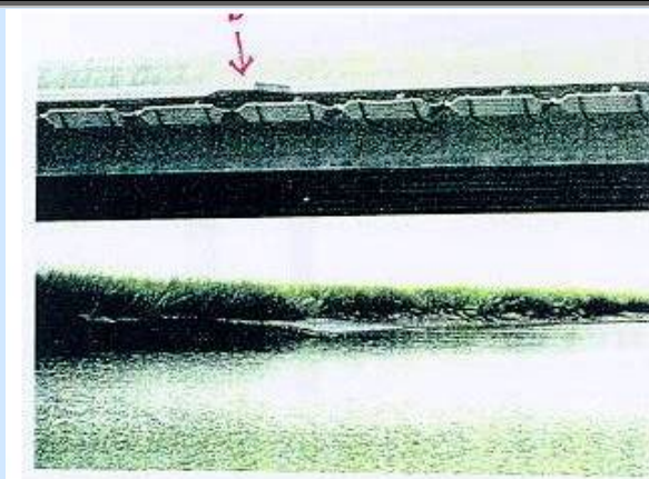
Figure 2.2-7: Stormwater pan system on the Isle of Palms Connector in South Carolina (Ross and Leitman, 1994).
